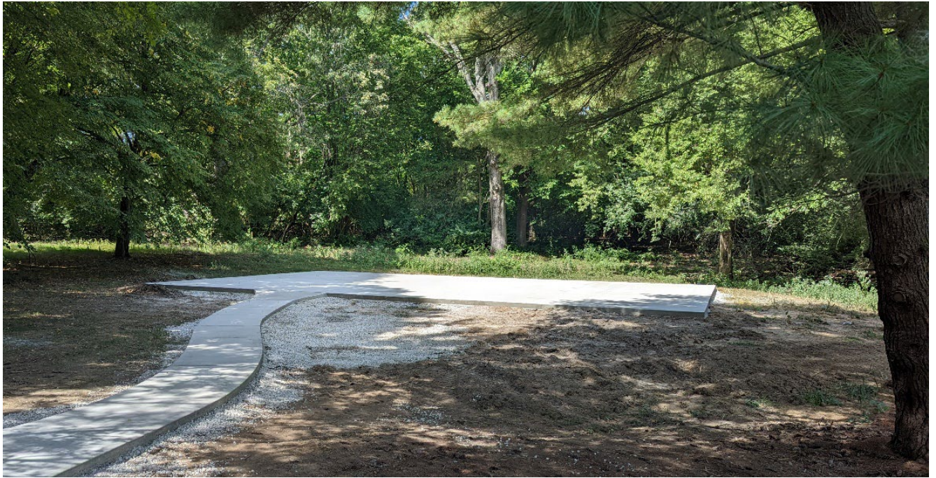
Concrete pad poured and setting up.
